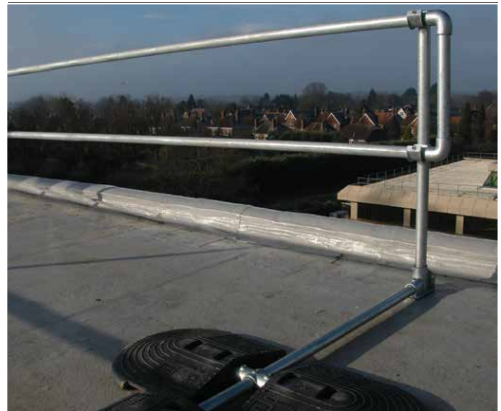
Alternative: KeeGuard counterweights can be used where returns cannot be used.
